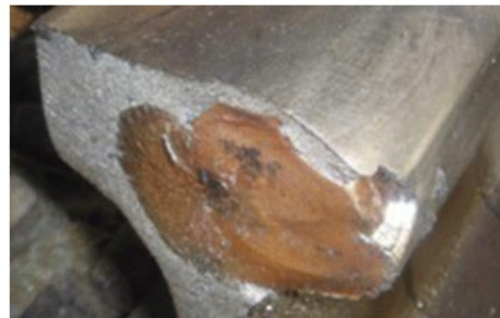
Figure 3: Transverse defect initiated by a deep seated shell from gauge corner collapse.
